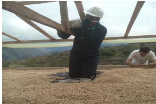
Fig. 12. Installing the radiation shield’s sensor.
