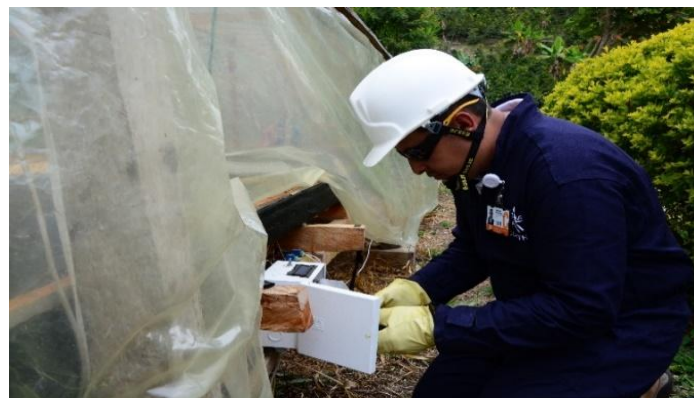
Fig. 13. Installing the whole system.
