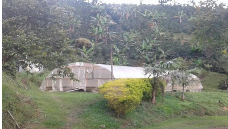
Fig. 11. System installed in “Mamola” coffee farm’s solar dryer.
